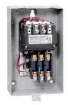
Non-reversing motor starter, Size 1 3/4, Three phase full voltage, Amb. compensate bimetal OLR, Contactor amp rating 40A, Non-combination type, Enclosure type 1, Indoor general purpose use
