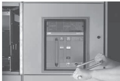
True Closed Door Draw out Capability
